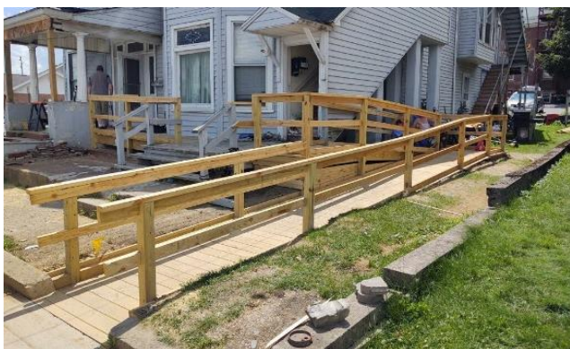
Completed ramp project
